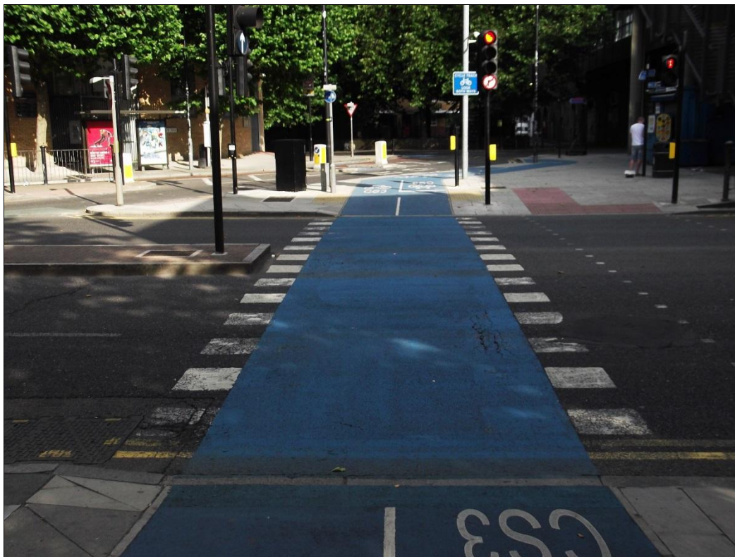
Example of a parallel crossing, Westferry Road, Limehouse
