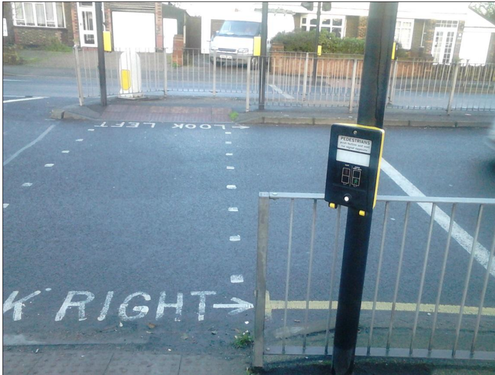
Main Road, southwest side of junction. Existing 2-stage, staggered PedX crossing (looking from south-eastern side to north-western side)
