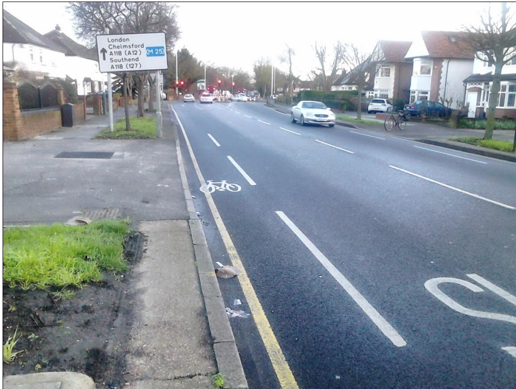
Main Road, southwest of junction. End of 1.1 metre wide advisory cycle lane 60 metres before junction.
