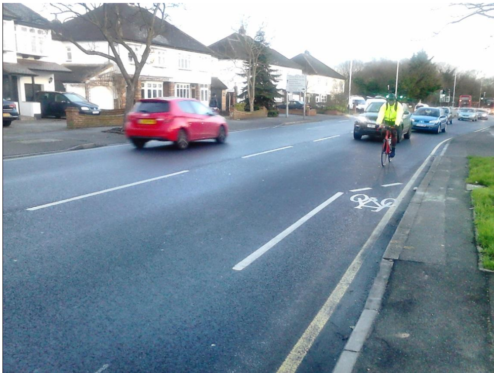
Main Road, southwest of junction. Start of Romford-bound 1.1 metre wide advisory cycle lane.
